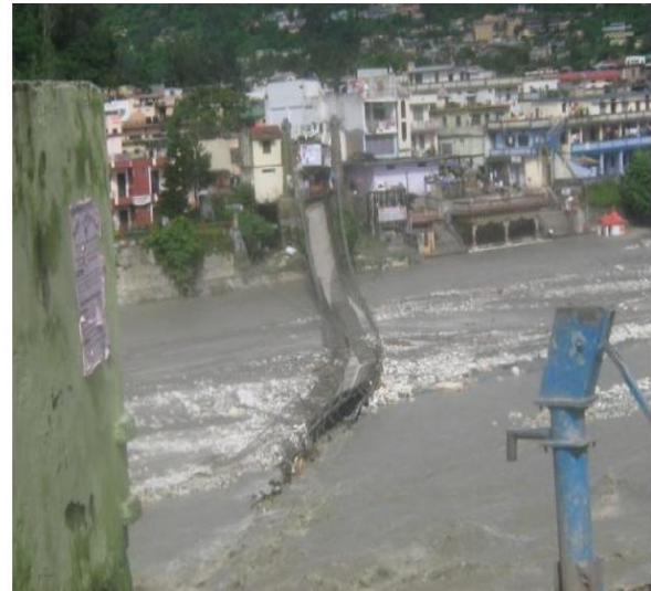
Figs 1.5: and 1.6: View of the bridges damaged by the flash flood in Uttarkashi.
